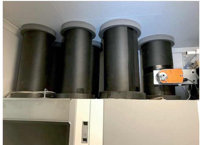
Cellular rubber insulated steel ducts
